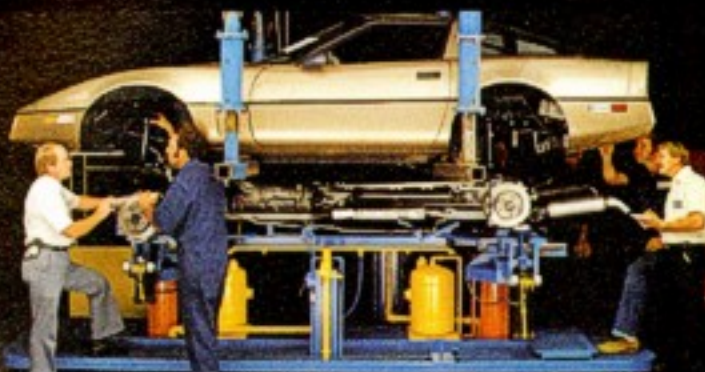
Specialty built hydraulic towveyer system "marries" chassis to body.
